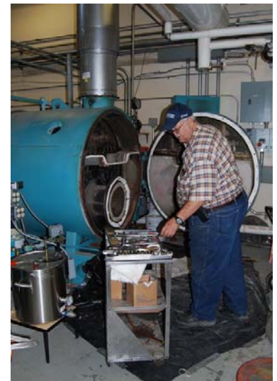
Building the cooking oil to fuel system
