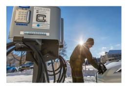
**Charger Specifications:** The Clipper Creek CS-40 Level II unit has a 32A (7.7 kW) charging amperage. Each charging cable is 25 feet. The station is UL-listed and works with all J1772 compliant vehicles.
